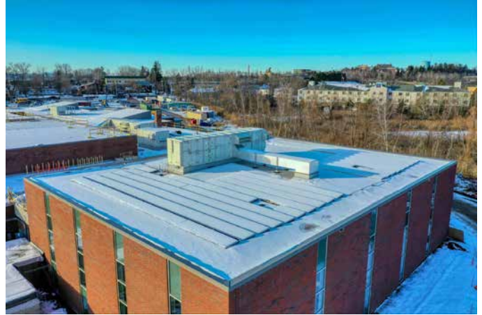
Photo of solar panels under the snow
