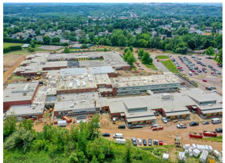
Building a better school - construction photo taken in July 2021.
