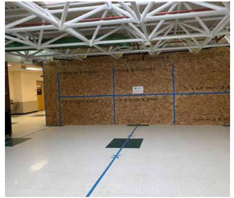
The construction wall where the new cafeteria will be located
