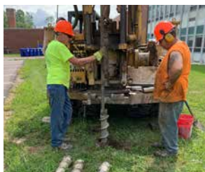
The drilling process.
